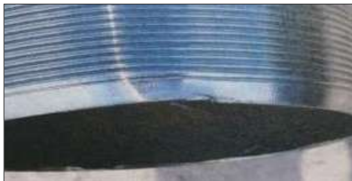
Photo. 6 Ding on the pin caused during transportation/
