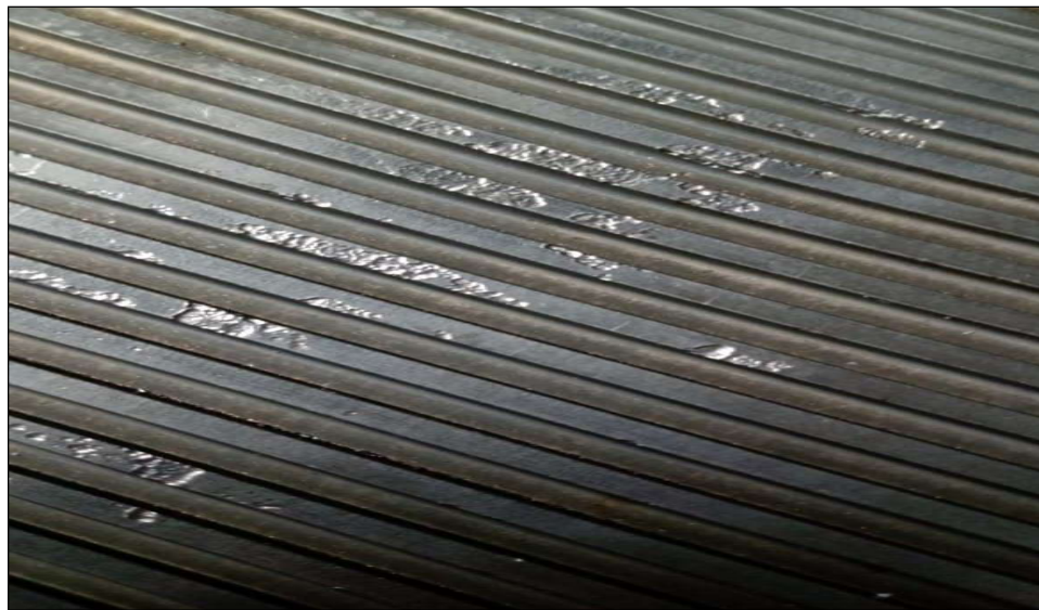
Photo.17 Major Pitting on a box connection; Rejected
